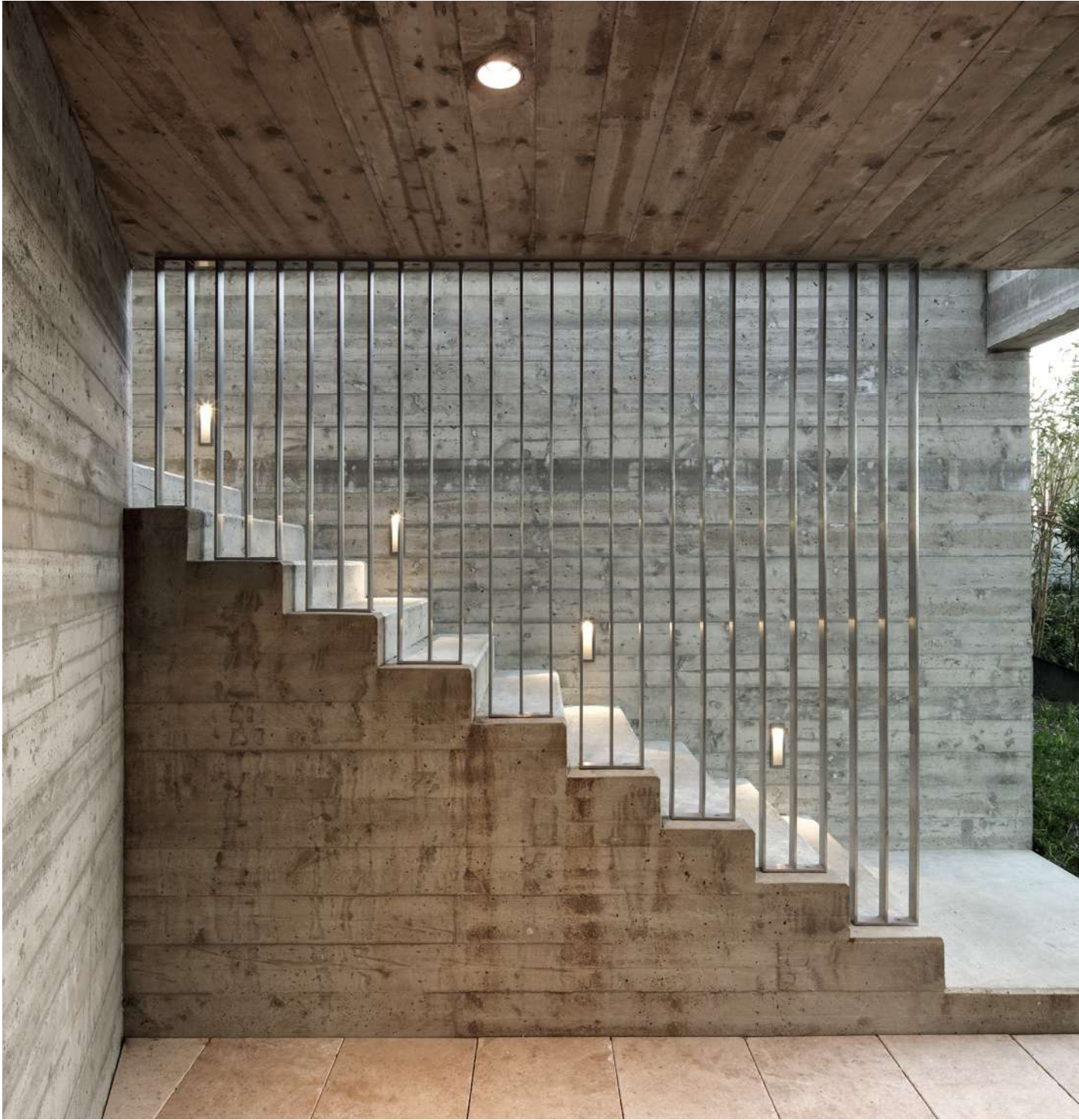
PRIVATE RESIDENCE | SPADO ARCHITECTS AUSTRIA
